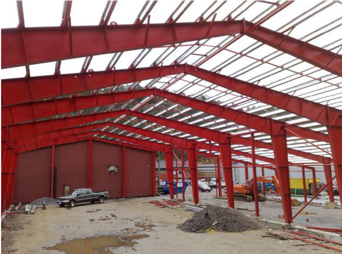
PTH provides detailed installation drawings and complete instructions for the installation of the joints of roof panels, walls, roofs and doors. In the installation of the roof, the length of the tiles exceeds 12 meters, and the disconnection design needs to be done. The project uses H-shaped steel, and there is no need to attach small steel on the side. Width to connect the upper and lower plates. This project is a hidden horizontal wall panel with no screws visible from the outside.
